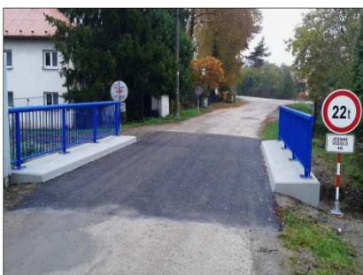
Mostek u sokolovny
